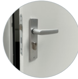
Wooden door frame and plywood entrance door
